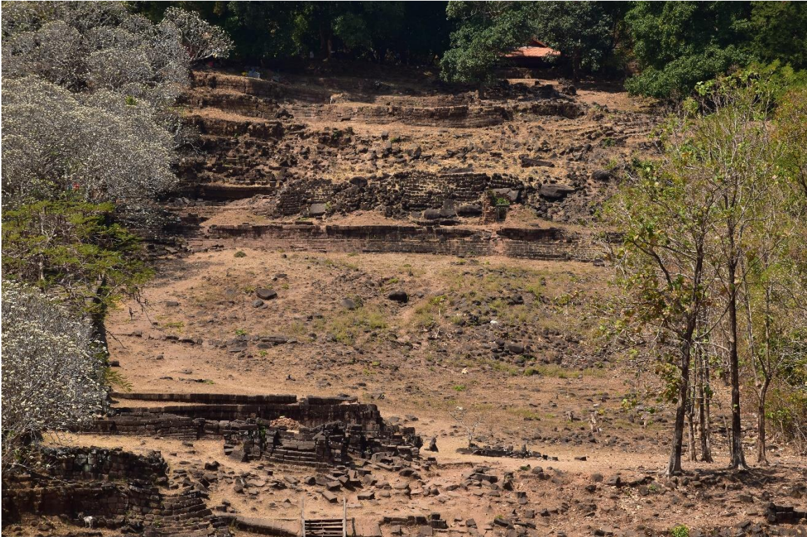
General view of 2 nd and 3 rd terrace
