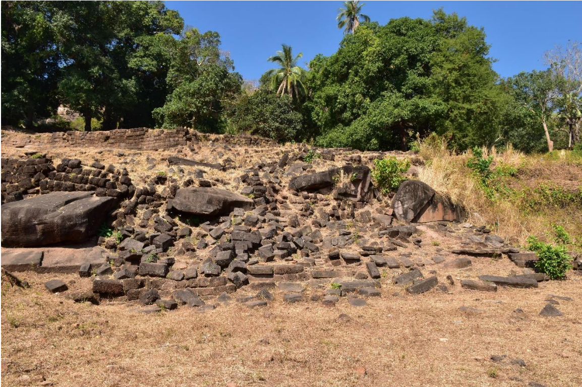
Fallen structures of 3 rd terrace
