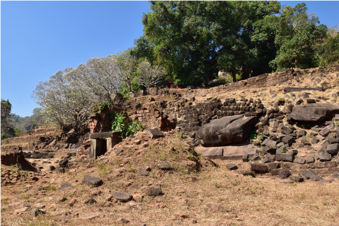
Fallen structures of 3 rd terrace
