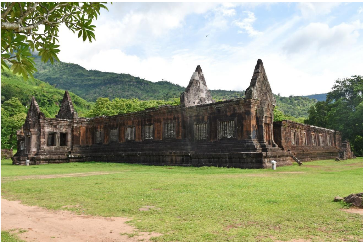
General view of Northern Quadrangle
